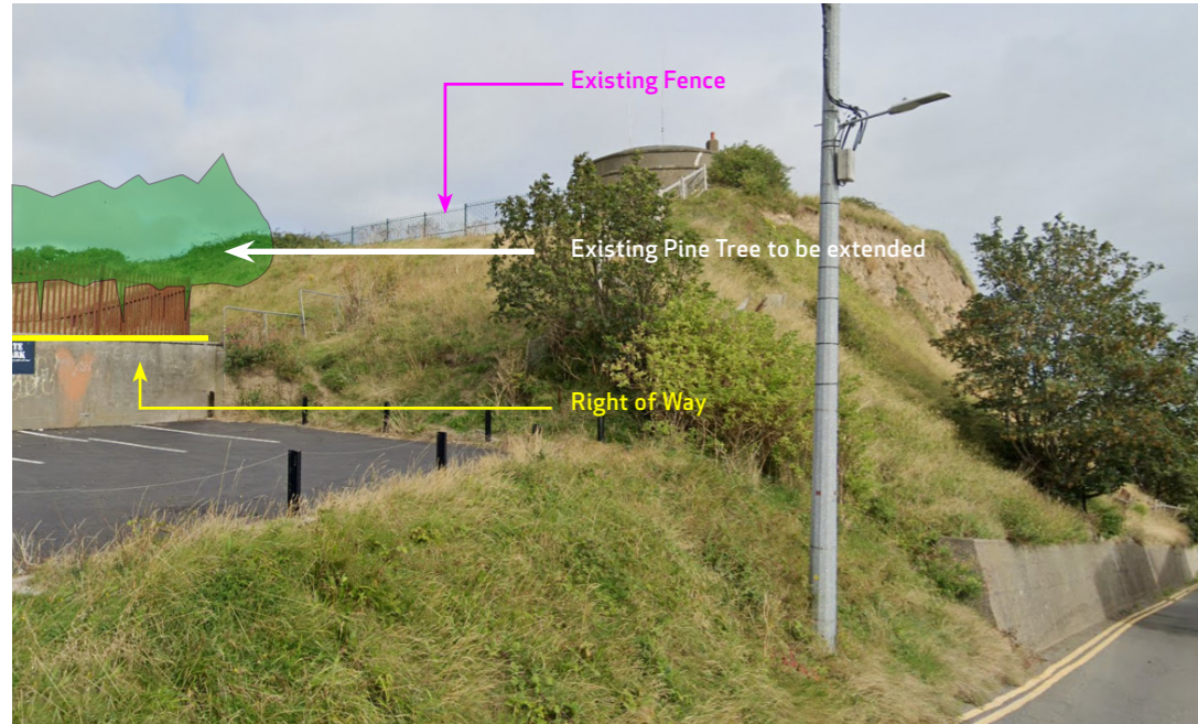
Embankment View from Balscadden Road
